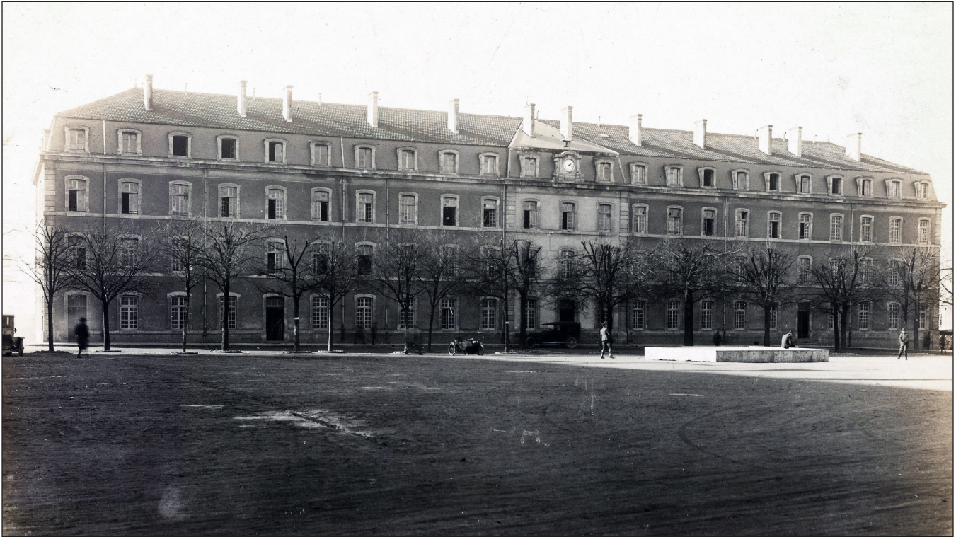
AEF Headquarters Building B, Chaumont, France. National Archives and Records Administration, College Park (NARA CP), Record Group (RG) 111, Records of the Chief Signal Officer. Photographic Collection, 111-SC-010062
