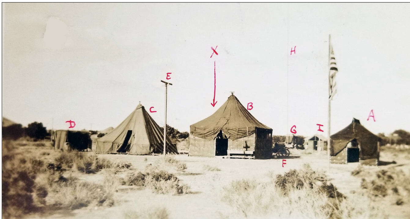
Radio Tractor Unit 43, Pecos, Texas, October 1918. A is the commanding officer's tent; B, enlisted personnel tent; C, supply and storage tent; D, gasoline, lubricating, and kerosene tent; E, electric power; F, Ford truck; G, tractor; H, 93-foot sectional antenna mast; I, operating house for cold weather; and X, the artesian well behind the tent. NARA CP, RG 165, Entry 65, Box 96
